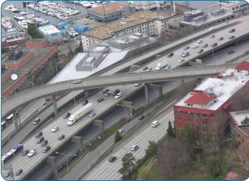
The I-5 express lanes at Lakeview Boulevard East
